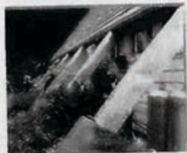
Before addition was built
