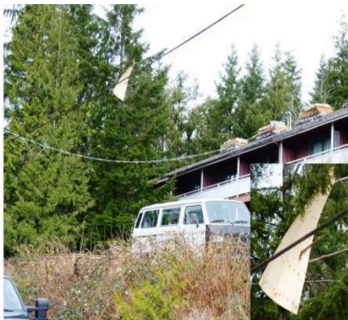
Wind rips 100 1/2-inch sheets of plywood off pub roof. One is impaled on a cedar branch. Photo M. Phillips
