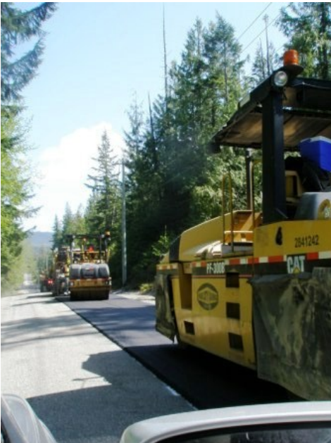
Black-topping the Bamfield Road. Only 74 km to go! Photo R. Hopkins
